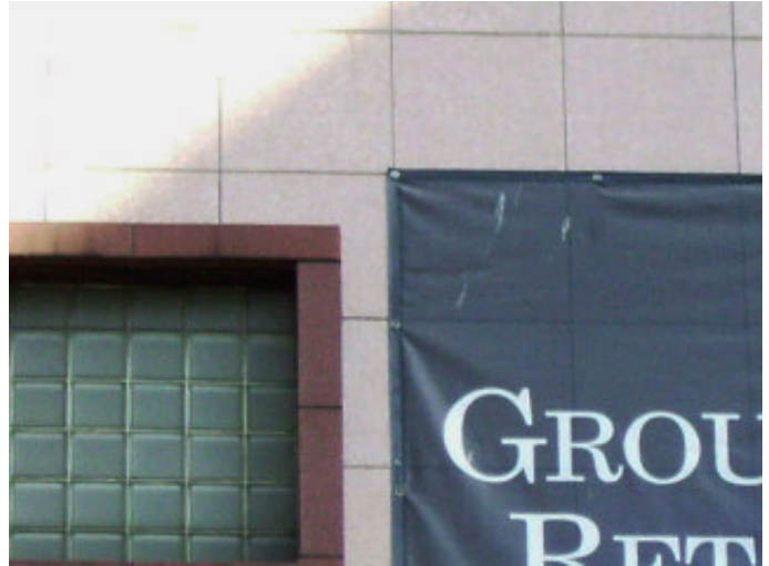
A clean installation using concrete anchors and washers into an edge reinforced with pvc-coated weldable webbing.
